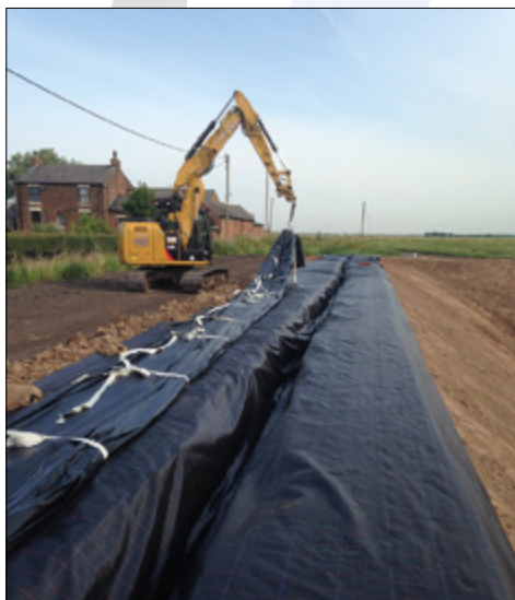
Protective sheeting laid over reservoir structure and liner pulled out.
