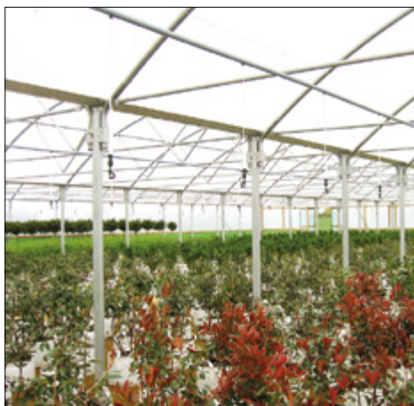
Overhead anti-drip spraylines.
