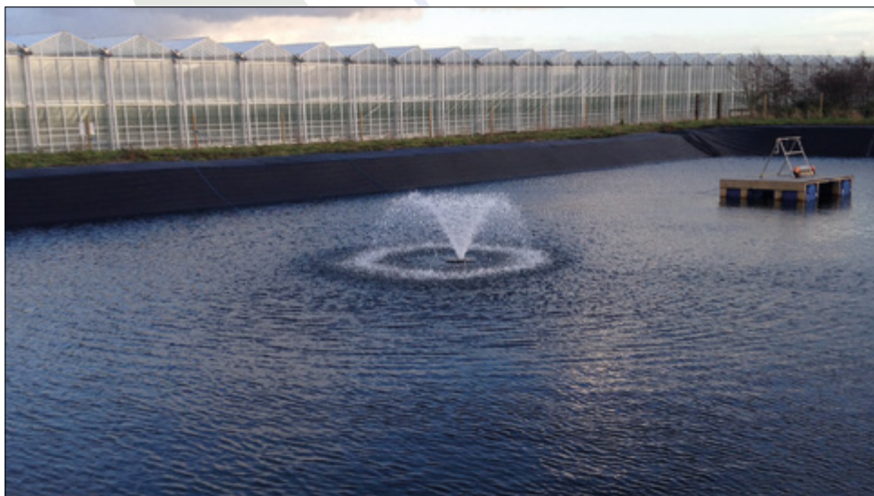
Finished reservoir with overflow and bank protection installed, aeration and pump transfer raft installed providing clear and uncontaminated water storage.
