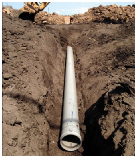
Overflow pipework installed providing maximum water retention.
