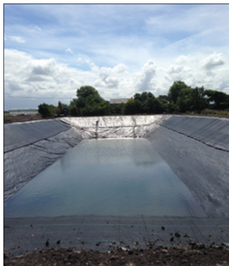
Reservoir liner dug in, bank protection sheet installed for sunlight protection.
