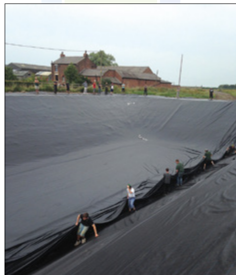
Liner positioned over protective sheeting and pulled up over all four sides.
