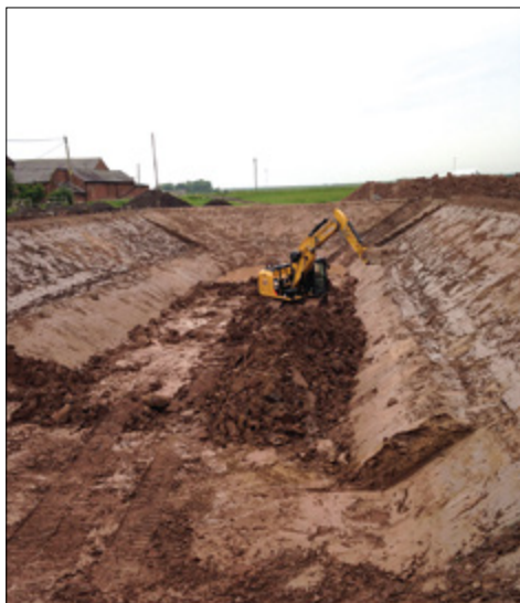
Profiling of the reservoir, angles checked with satellite measuring.
