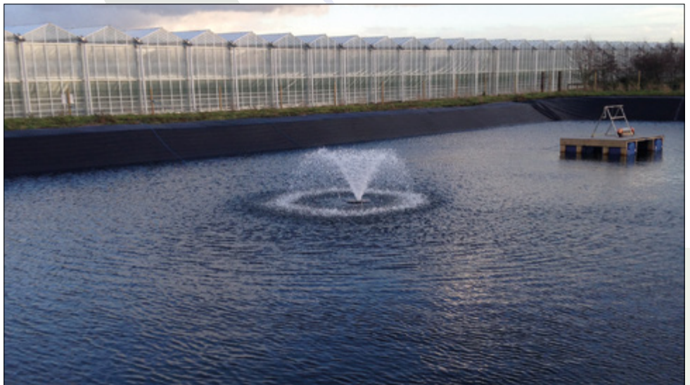
Finished reservoir with overflow and bank protection installed, aeration and pump transfer raft installed providing clear and uncontaminated water storage.
