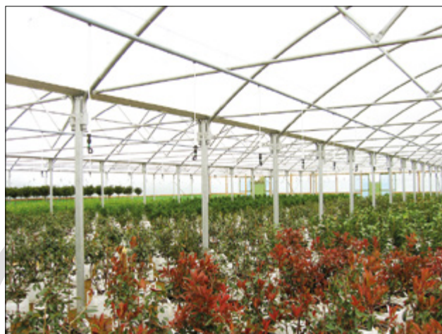
Overhead anti-drip spraylines
