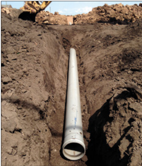
Overflow pipework installed providing maximum water retention.
