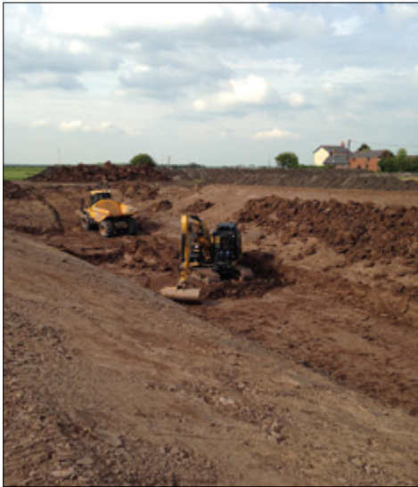
Removal of clay to create depth and reservoir banking.
